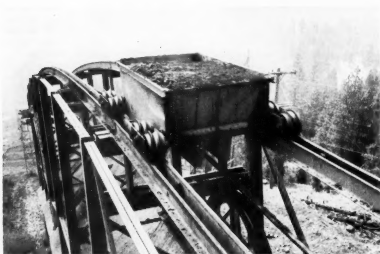
TRAM CAR containing 2½ tons of nickel ore starts trip down 8,306 foot long aerial tramway which has a rated capacity of 250 tons an hour.
